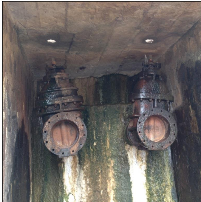
Figure 5 Bindangombe dam outlet works
