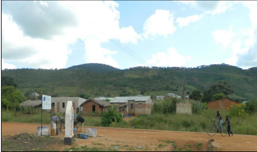
Figure 10 Low cost or rural housing units at Mwami Border Post
