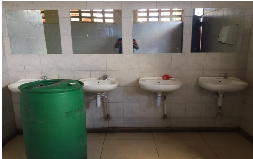
Figure 2 Wash basins in the Passengers Terminal Ablution Block
