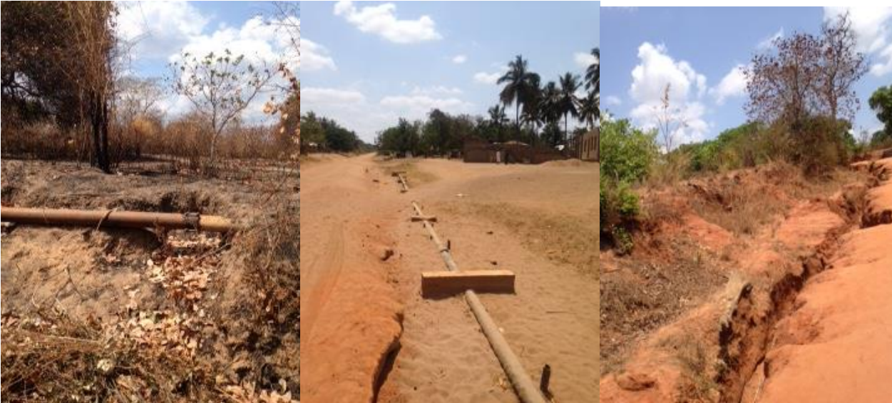
Figure 21 Erosion in the project area
