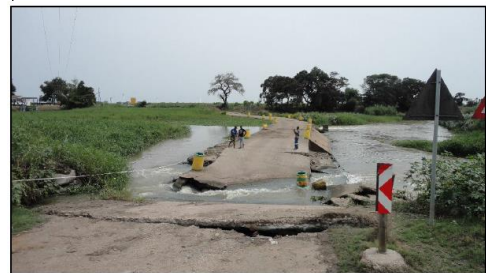
Figure 7-8 Flow Comparison over the Weir by Xinavane Mill for the 1 in 10 Year Flood Event, the photograph was taken during the CRIDF topographical survey.
