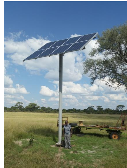
Figure 2: Typical solar panel for motorised borehole in Hwange National Park
