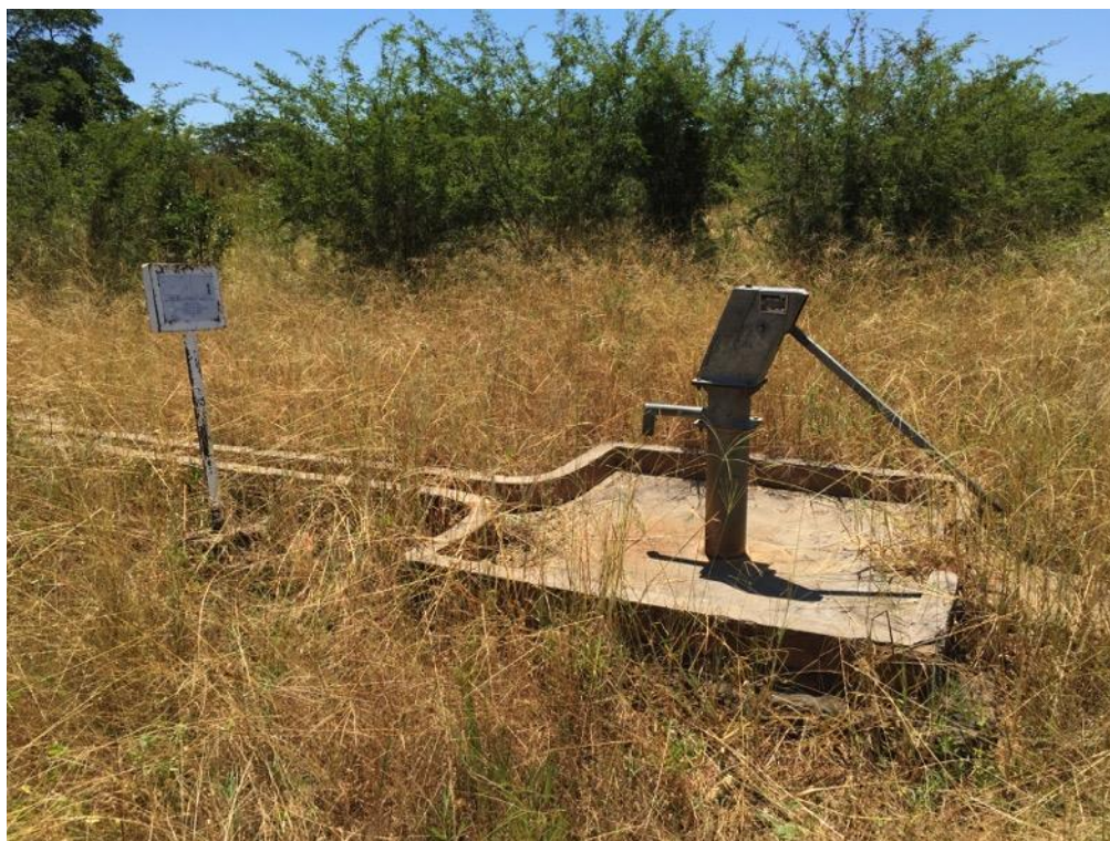
Figure 5 Non-functioning borehole, Namuse
