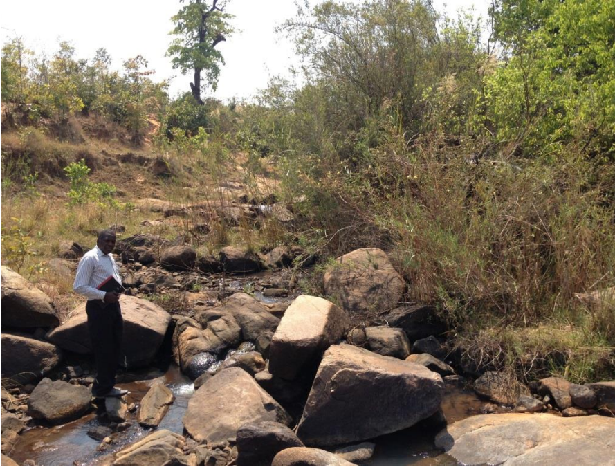
Figure 5 Pick-up weir site
