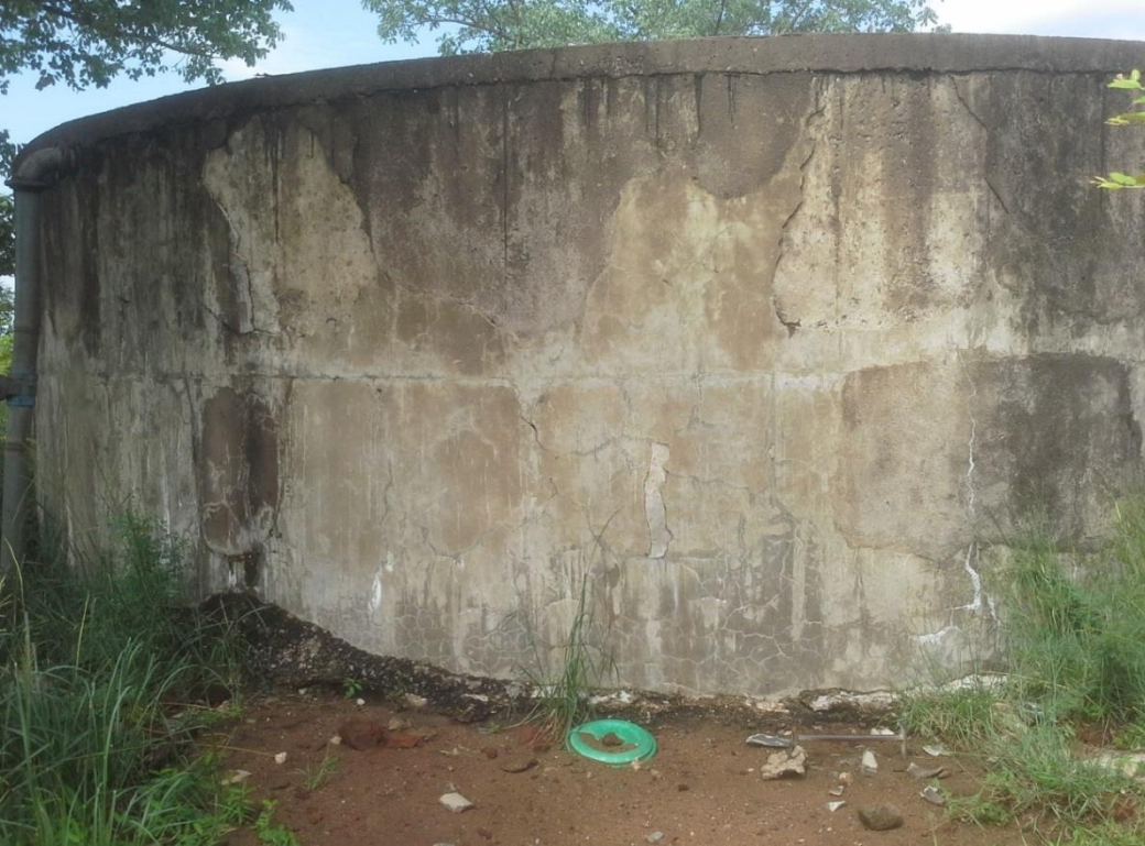
Figure 7: 200 cubic meters existing concrete tank
