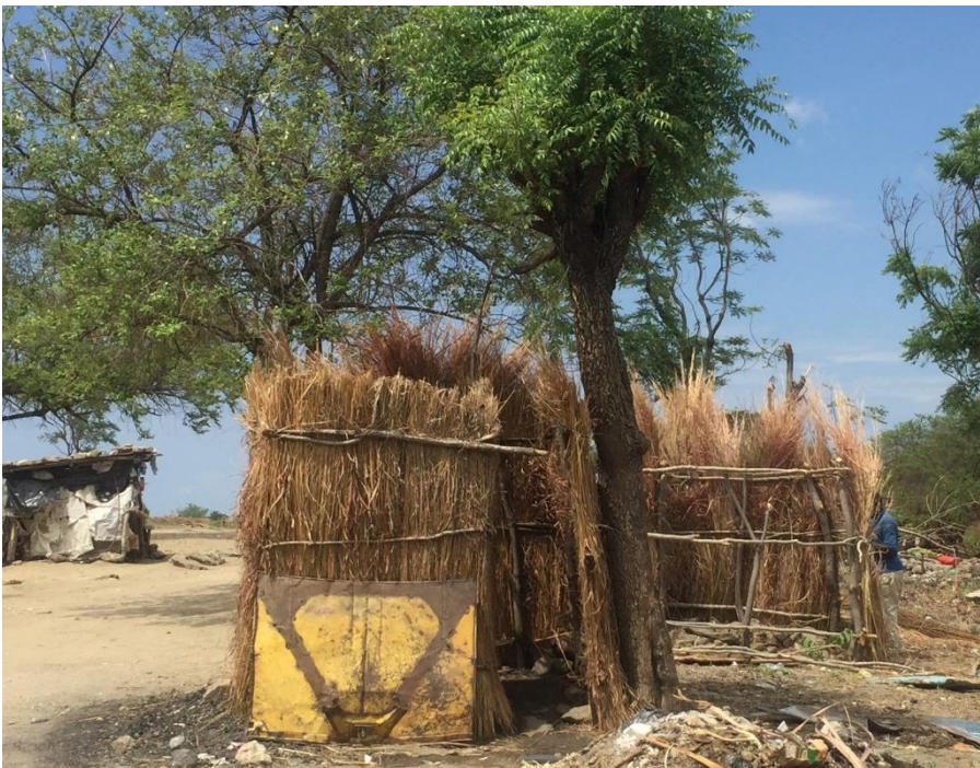
Figure 11: Poorly constructed latrines in Micho Settlement
