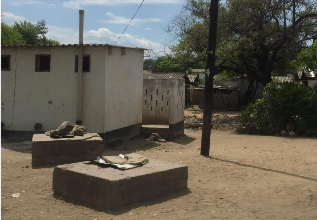
Figure 9: Communal ablution block and septic tanks
