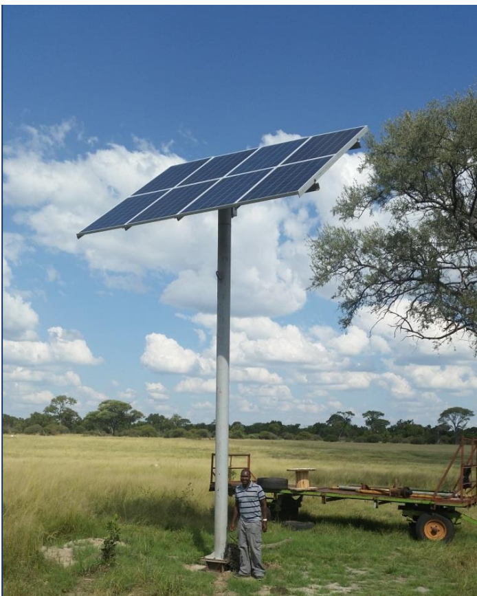
Figure 5: Example of solar pump used in the KAZA Zimbabwe area
