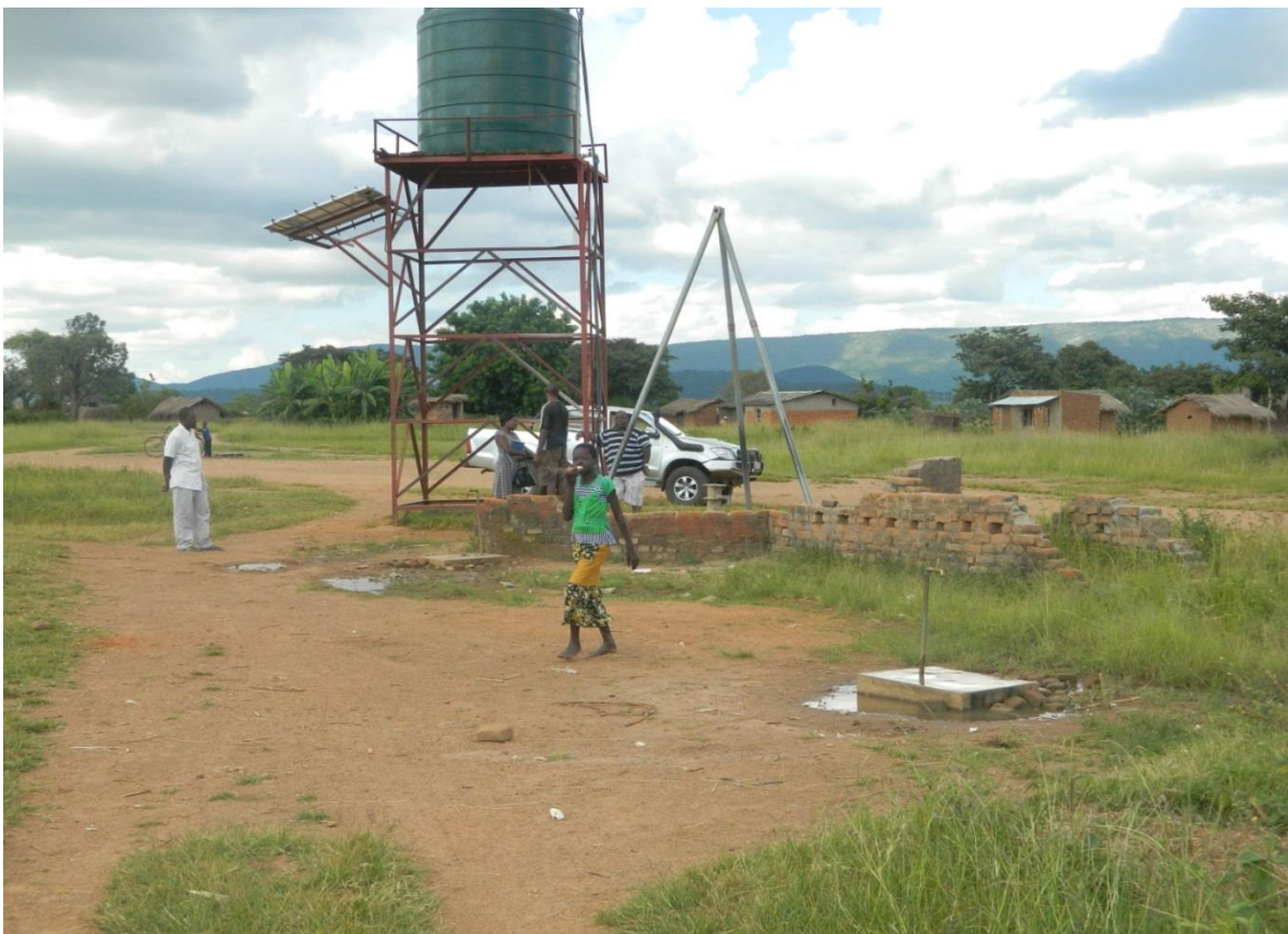
Figure 7 Sanitary conditions around the taps at MWA002
