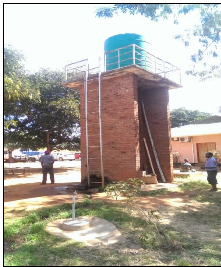
Figure 9 MRA Borehole and Elevated Tank
