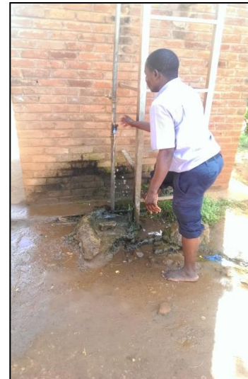
Figure 10 Standpipe at MRA Tank
