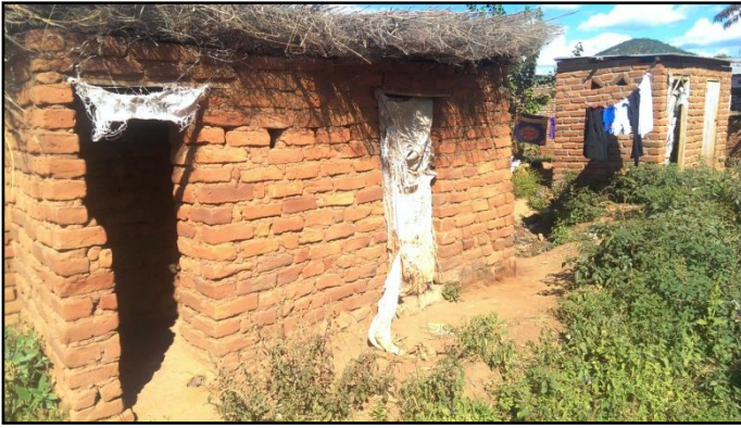
Figure 11 Pit Latrine Top Structure
